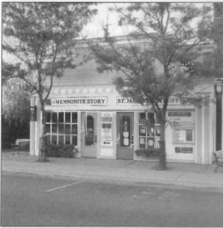
The Mennonite Story building as it looks today in downtown St. Jacobs. Photo courtesy of St. Jacobs Printery.
