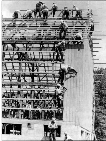
This 1977 photo shows the many hands needed to complete the job. Photo credit: Mennonite Archives of Ontario/K-W Record (Gerry Bookhout)
